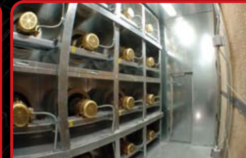
16 fans per fan wall per unit producing 75,000 CFM at N+4 per TSC
