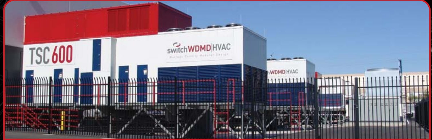
Quad Process HVAC Units - WDM | TSC 600 Tons Each
