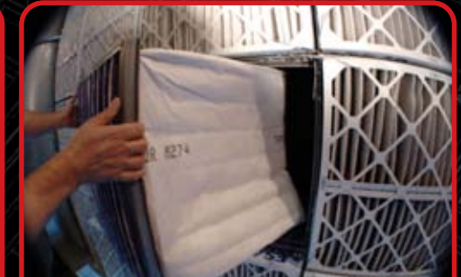
Dual box and bag filter zones allows up to MERV 20 filter rating for outside air
