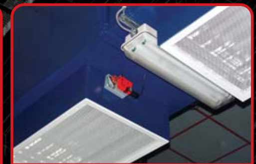
Automated damper controls for real-time CFM adjustment by L.D.C.
